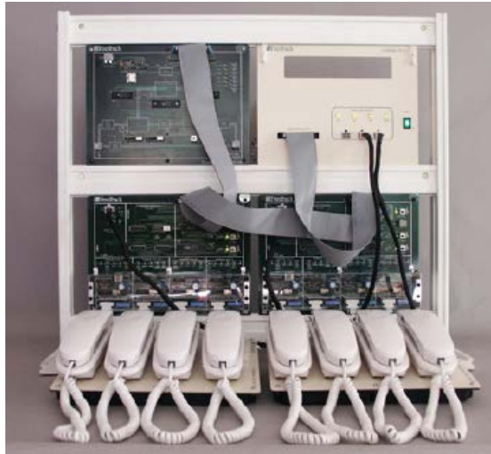
Fig. 4. The whole Digital Switching system.
